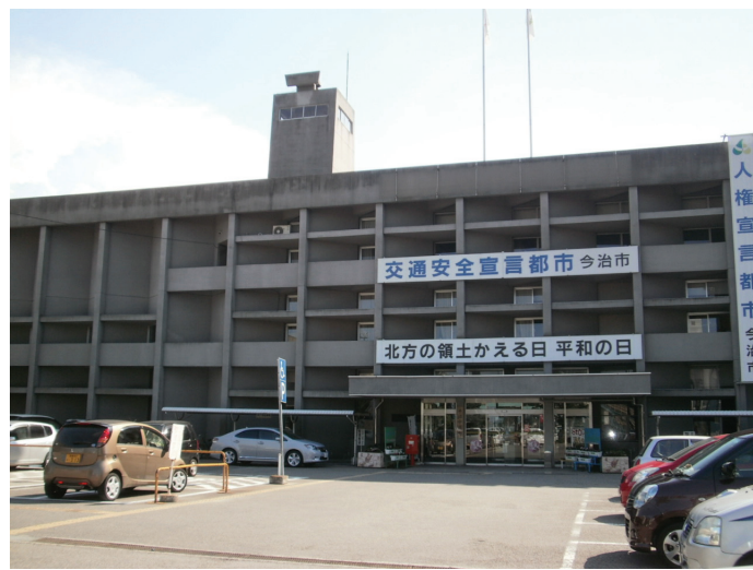
Imabari City Office (今治市役所)
